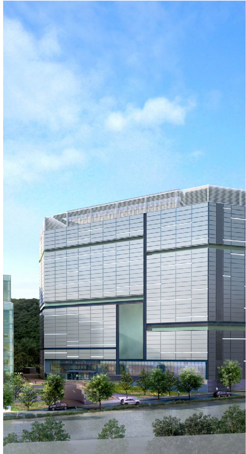
Empyrion data center in South Korea
