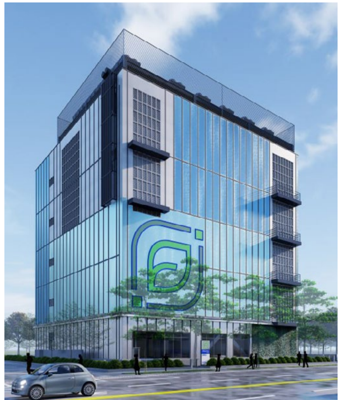
Empyrion data center in Taiwan
